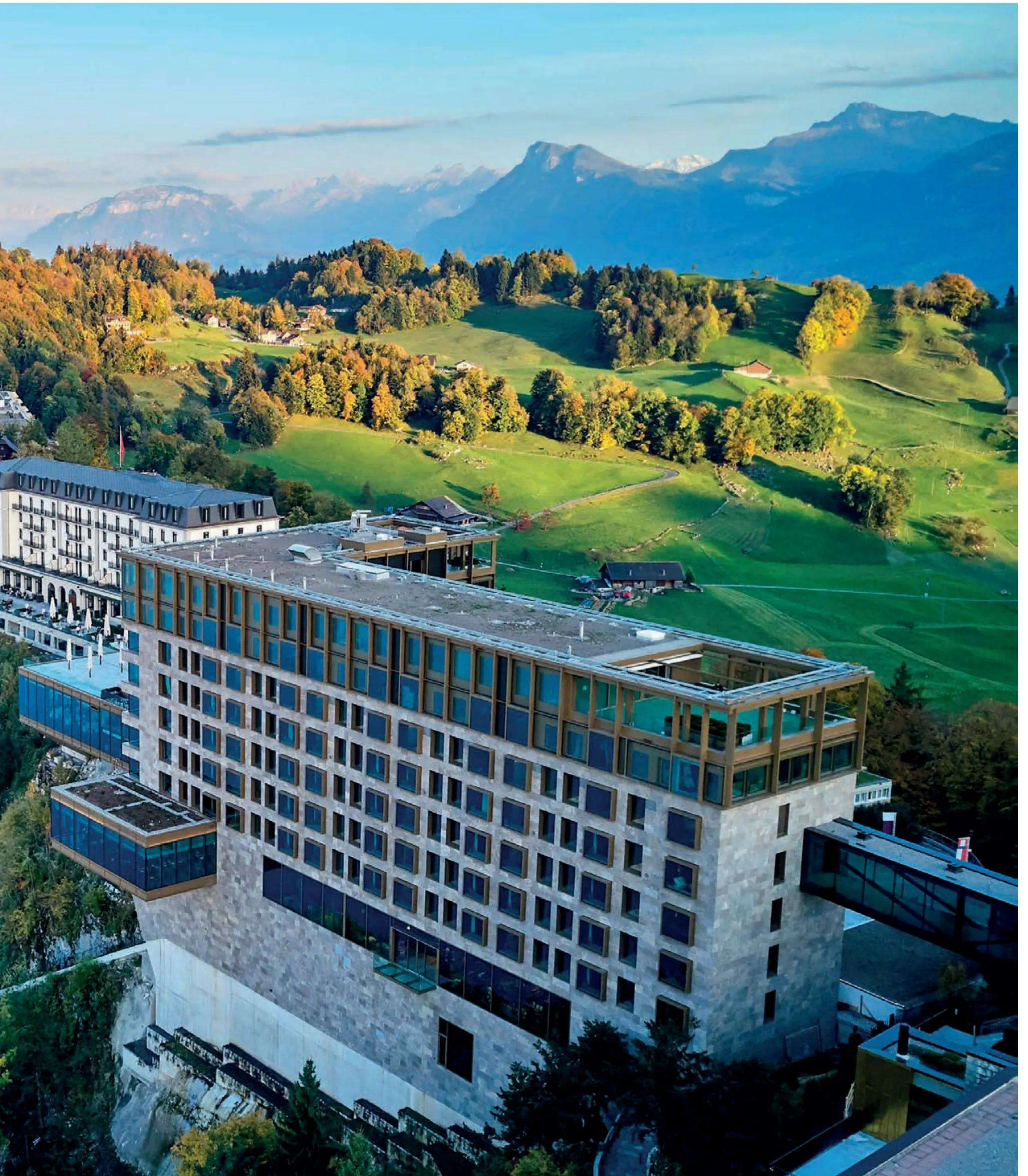
Bürgenstock Hotel & Alpine Spa
